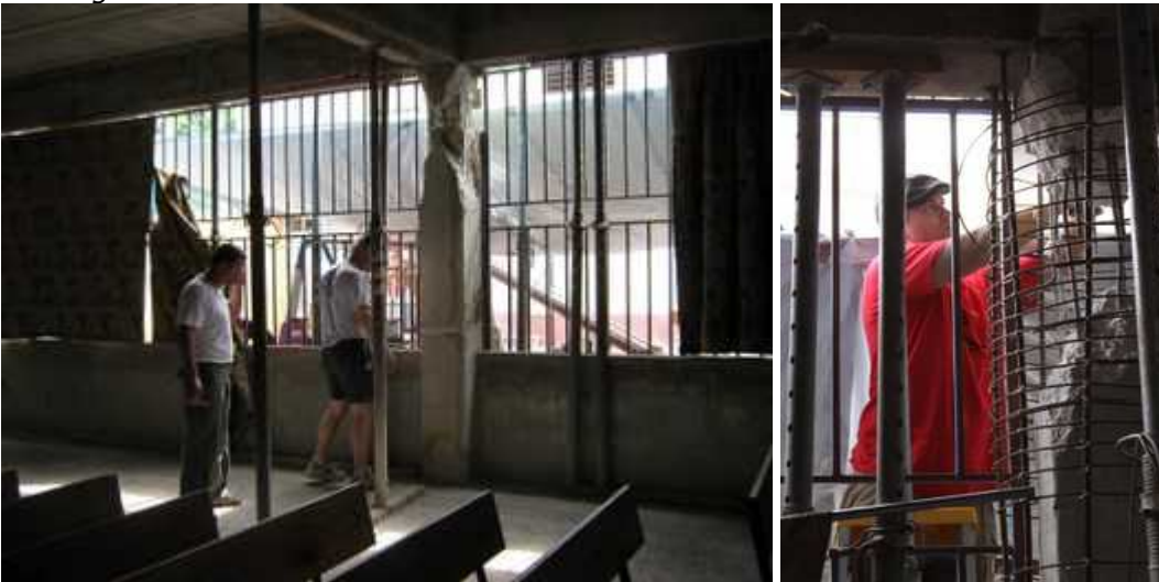
Working on a column in the church
