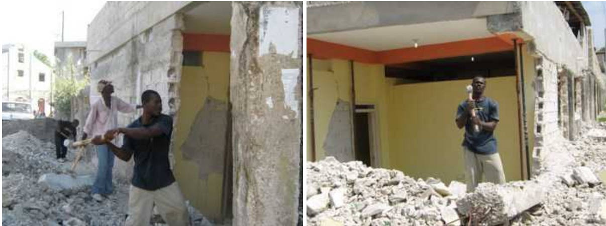
Demolishing a portion of the damaged perimeter wall
