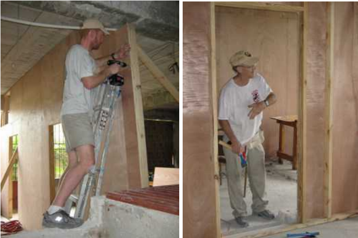
Working on the new Media Room
